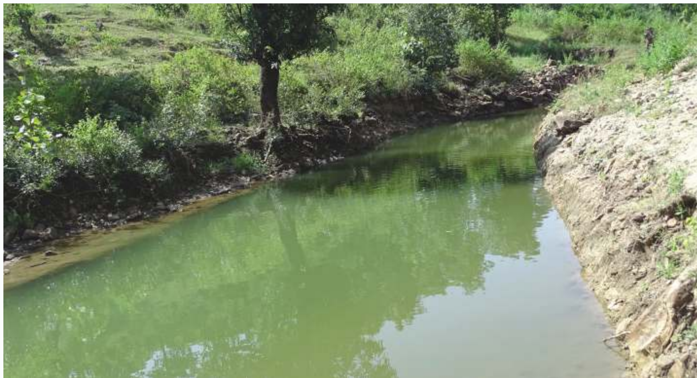
A "DOHA" in village Jamli, Chicholi block of Betul district, Madhya Pradesh. ASA has initiated DOHA model- low cost water harvesting structure build on the stream bed to augment water recharge. 13 Dohas have been created irrigating 20 ha.
