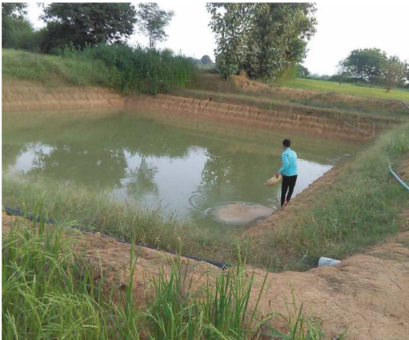
Farm pond constructed in village Umriya by Smt. Mamta bai in Mehandwani district. They are also experimenting by sowing fish seedlings.
