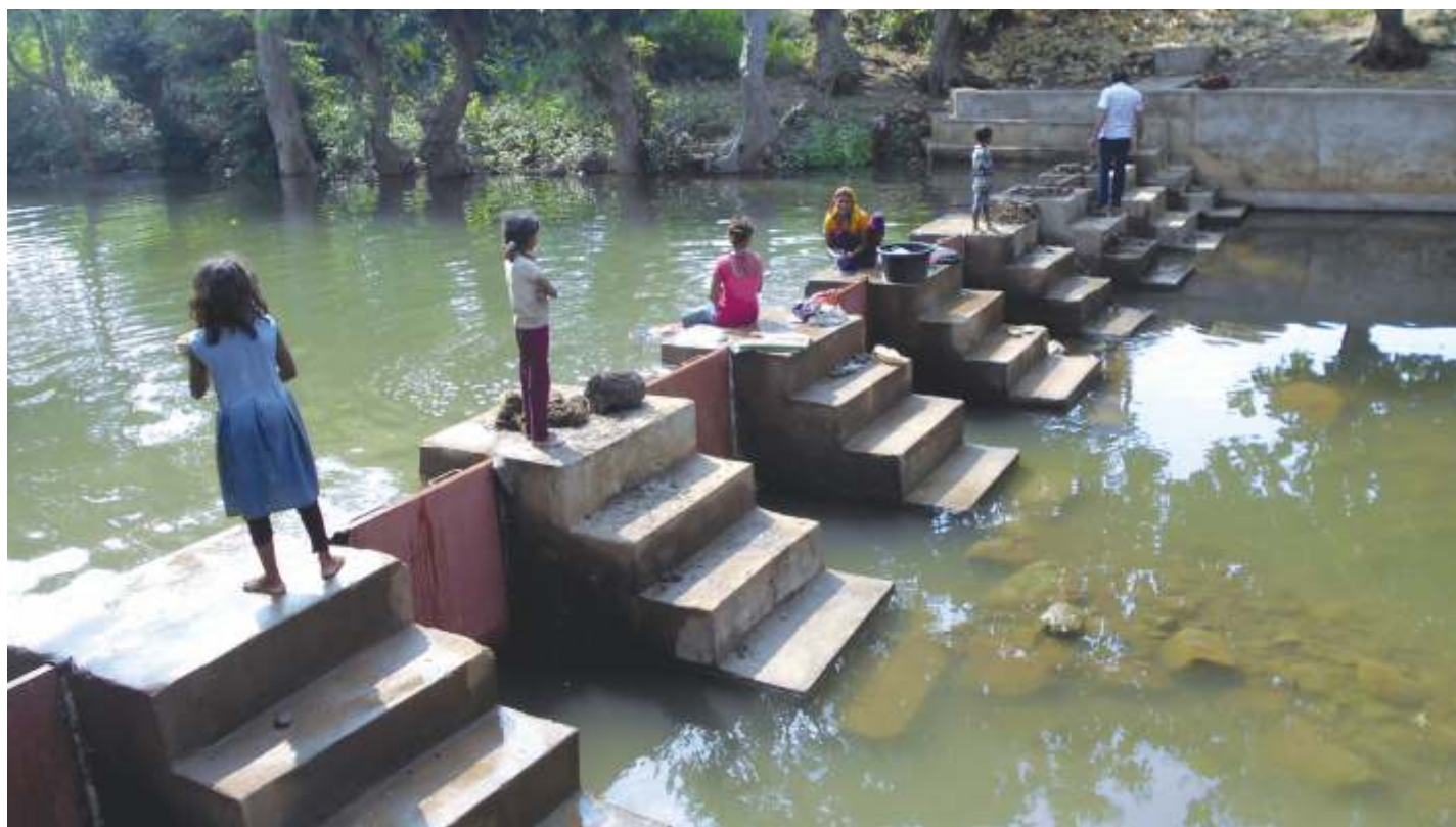
Stop dam in village Bela, Chicholi Block, Betul district, Madhya Pradesh.
