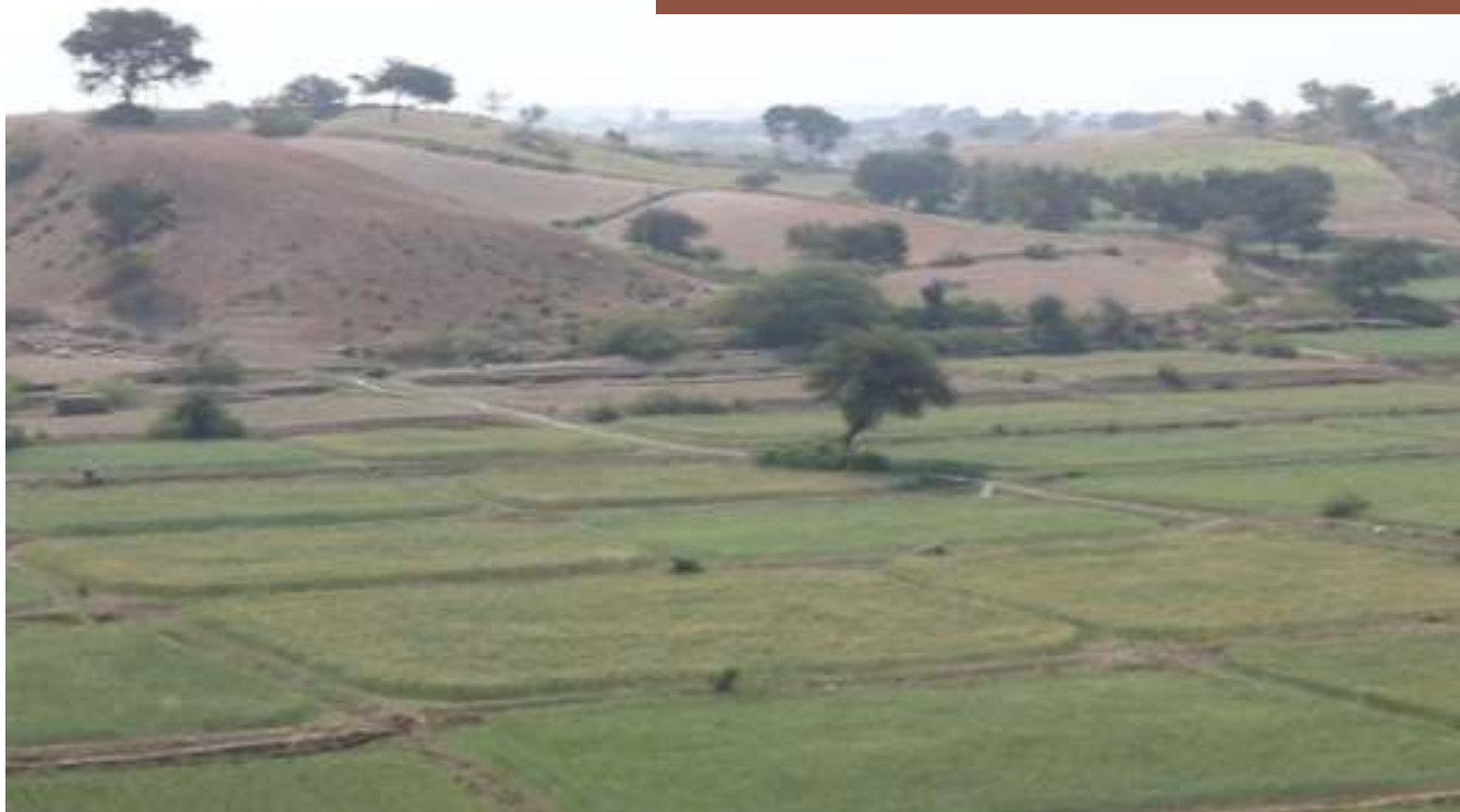
Bird's eye view of irrigated fields from masonry stop dam build more than 10 years back in Ranapur district, Jhabua, M.P, being independently managed by the Water User's Group.
